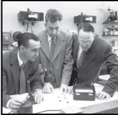
The inventors of the Bell Solar Battery, from left, Gerald Pearson, Daryl Chapin, and Calvin Fuller, check devices for the amount of solar electricity derived from sunlight, here simulated by a lamp.
